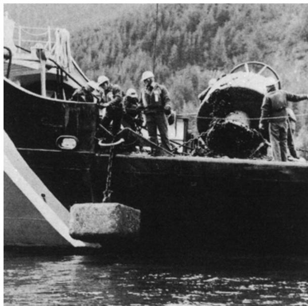
Figure 512. A sinker used to anchor a buoy.
