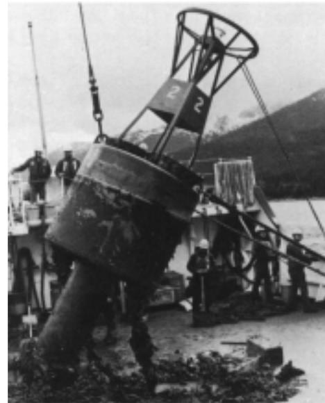
Figure 509. Buoy showing counterweight.
