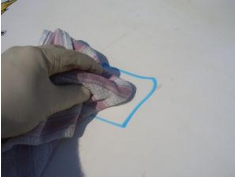
Clean off the sanded area with alcohol again, to make sure there's no grease on the surface.
