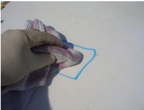
Clean off the board's surface all around the hole, using a rag soaked in alcohol.
