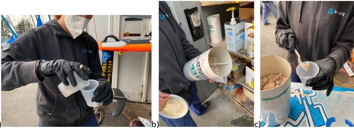
Figure 5. Adding filler to the epoxy to increase viscosity a) split your dose of epoxy to have some pure epoxy later on. b) The filler is in the closet. c) Progressively add filler to the epoxy until you get a viscosity close to peanut butter
