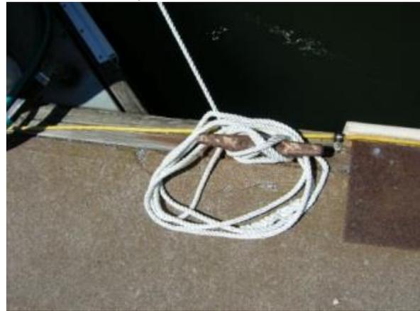
Why: A jumble of line creates a tripping hazard. The lines can get kicked into the water, and they can get stepped on, too, which is not good for the line.
